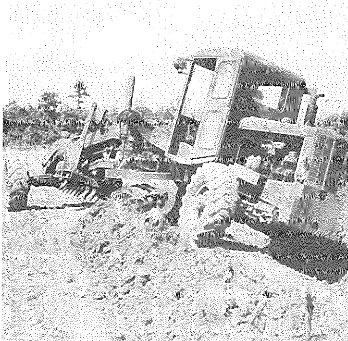
13. THIRD PASS, OR WINDROW MOVE-OVER.
