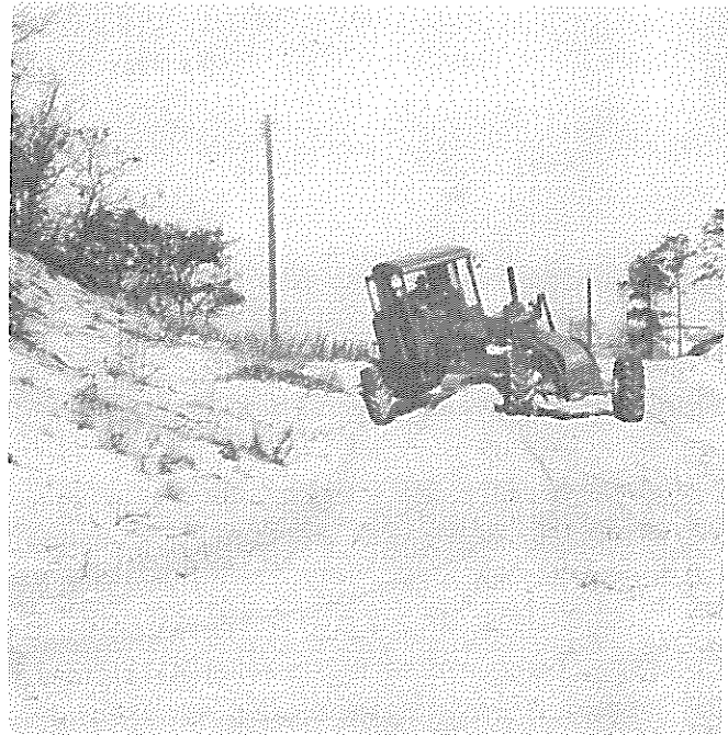
14. WINDROW MOVE-OVER IN BLOW SAND.
