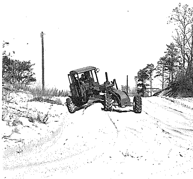
8. WINDROW MOVE-OVER IN BLOW SAND
