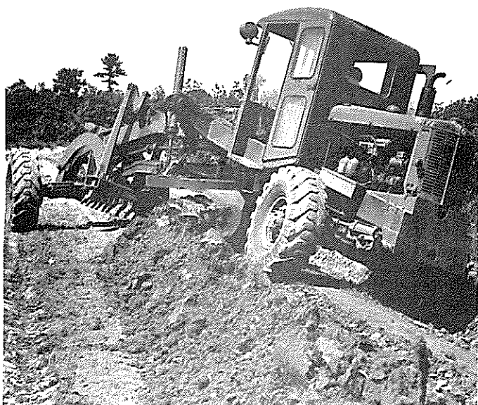
7. THIRD PASS, OR WINDROW MOVE-OVER.
