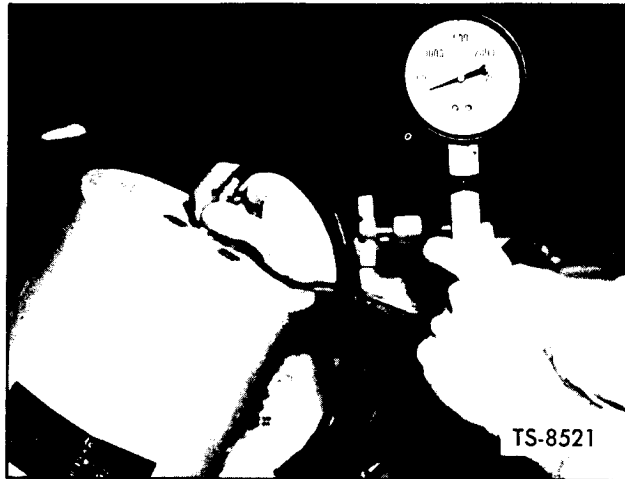
Fig. 22. Checking Accumulator Pressure
