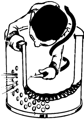
Blowing out dust with compressed air.
