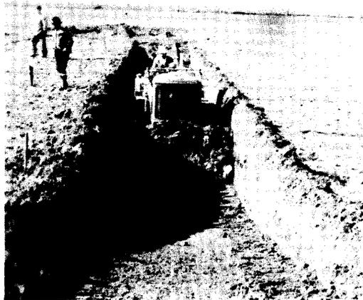
At the end of each pass the tractor is reversed and backed through the trench rather than turned around unless it is desirable to push material from each end of the trench.
