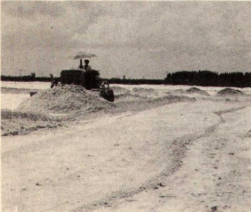
Some material can be levelled off by dragging the blade while backing up. It is much easier for the beginner to finish in this manner. Anything which speeds up any operation makes it just that much easier and more efficient.
