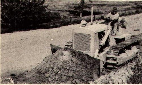
If the ground is very uneven, it will be necessary for the operator to first level a small place from which to start operations. Always start cutting when the tractor is level or from this initial starting point. Do not start cutting when the tractor is tilted to either side because the farther the tractor travels ahead the more it will tilt and the more
