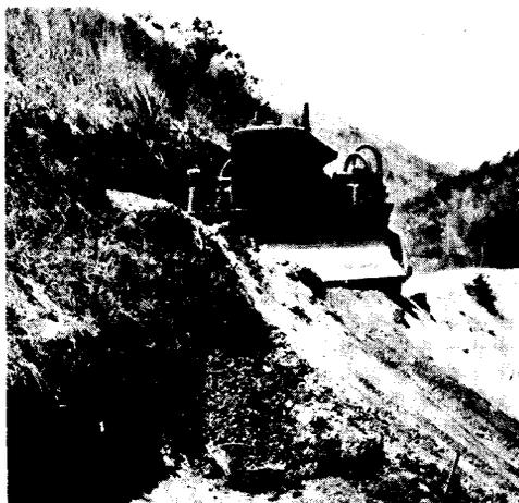
To get full efficiency from the tractor it should be kept as nearly level as possible and worked downhill as much as the job will permit.
