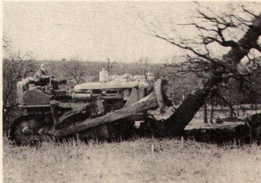
making contact and try to have the tractor on good footing, so the thrust will fall the tree out of the right-of-way and not on trees to be cleared later. The trees when felled will push into the nearby forest easier lengthwise than crosswise.
