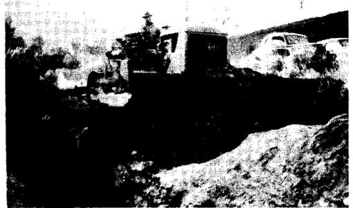
has been cast on both sides of a ditch, it will usually be possible to backfill it by making a pass on one side, returning down the other side for one pass and completing the filling with a final pass on the first side. This avoids changing the blade angle. Any length ditch may be filled in this manner.
