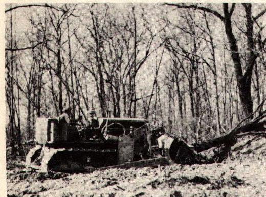
In clearing, if trees are to be removed, the tractor should start at the lowest point to be cleared, unless it is possible to push all the material in one pass with the machine. With the blade angled, drive up to the tree in low gear and make contact easy. Do not strike the tree at high speed as the top of the tree may break out, damaging the machine or injuring the operator. Nothing is gained by this type of work. Place the blade high on the tree in
