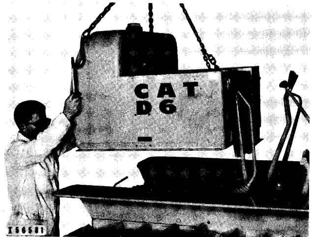
REMOVING FUEL TANK
