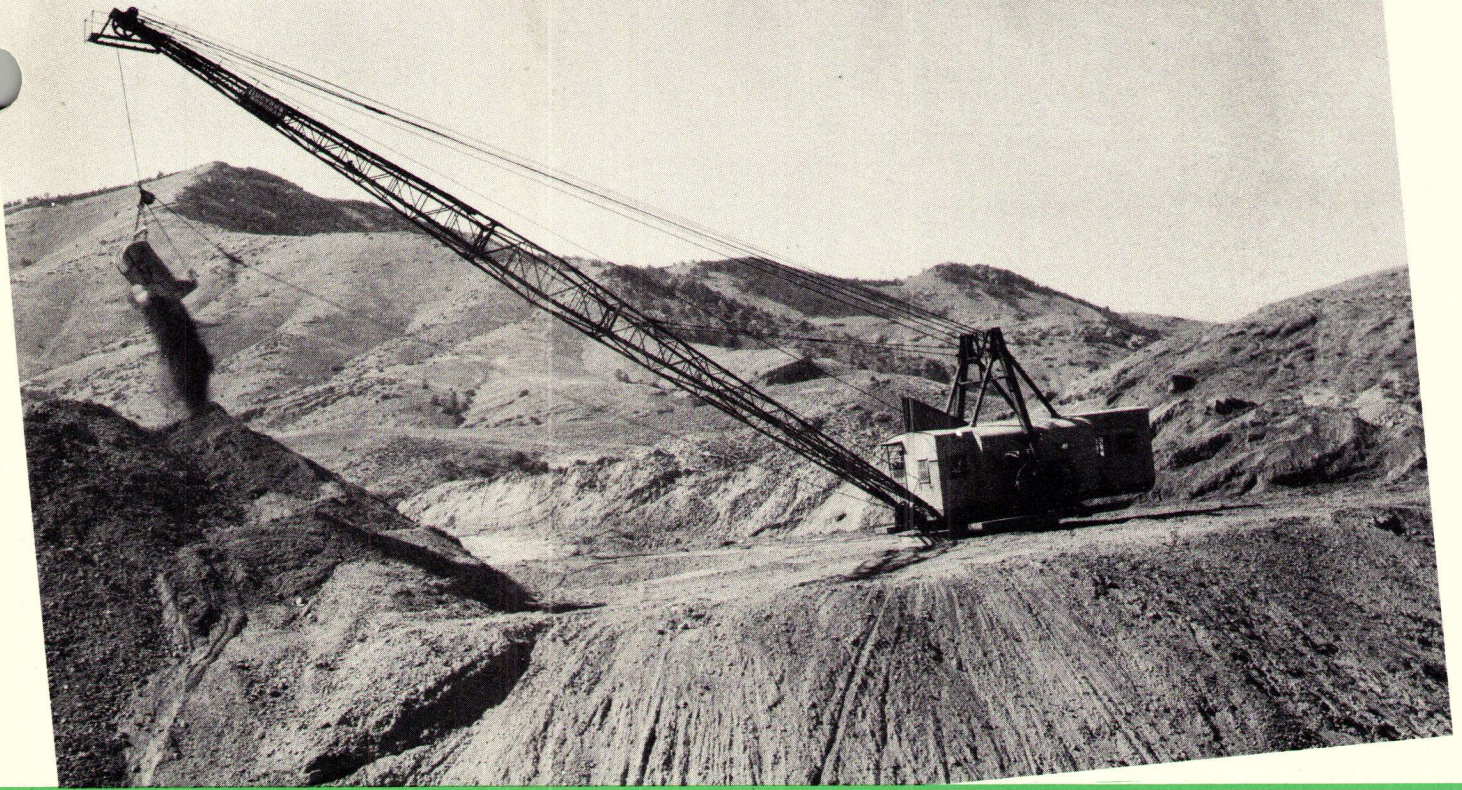
Ralph E. Davis uses this 5-W with 125-foot boom and 4-yard bucket on a drag-line-dredge gold-mining operation near Dillon, Montana.
