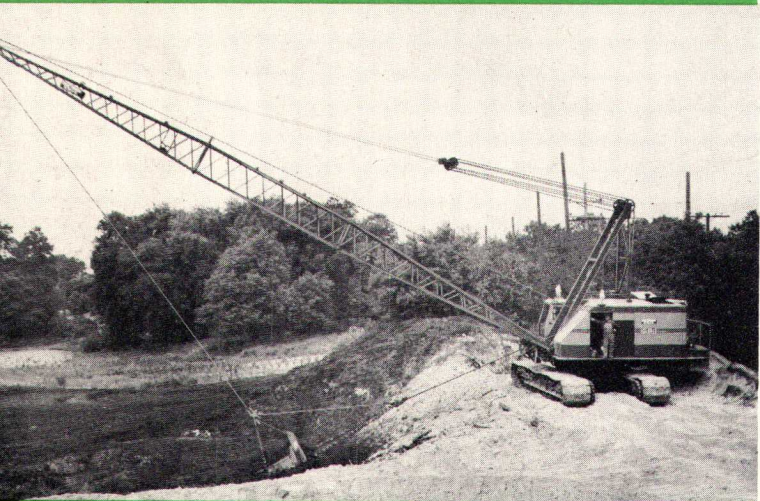
Calumet Paving Company's 54-B replaces muck with dry fill on highway job.
