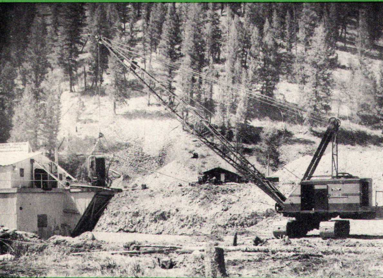
J. L. Shiely's 54-B dragline loads gold-bearing gravel to a hopper in Montana.
